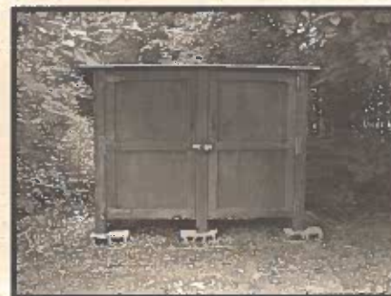
Lunch Box Storage Container, constructed by Tony Lyon Loftus. This structure houses student's lunches while they are at Renfrew for day-long Institute programs.
