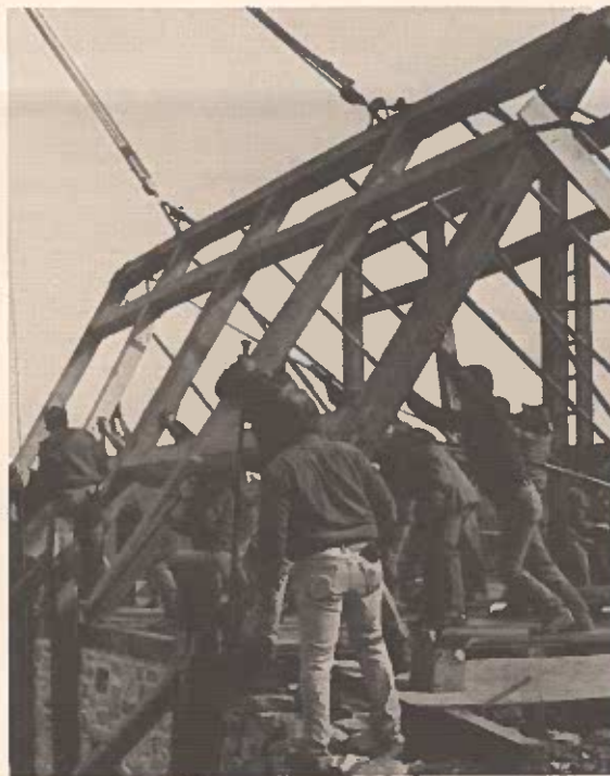
Raising the west bent of the Fahnestock barn Photo - Bonnie Martin The Record Herald
